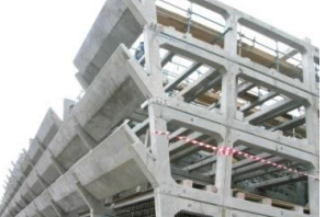
Drajat Cooling Tower – Garut (2005) Thiess*
