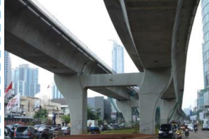
Overpass Kamp. Melayu – Tanah Abang (2014)
