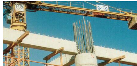
Precast walls, columns, beams, stairs and other structural and architectural components.
