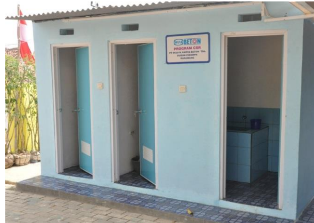
Sanitary facilities for public
